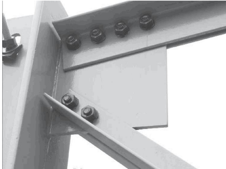
Figure 6.9 Typical bolted truss and gusset plate connection
