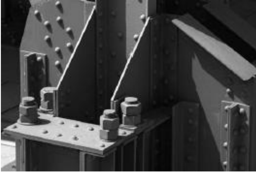
Figure 10.19 Typical application of bolted connections
