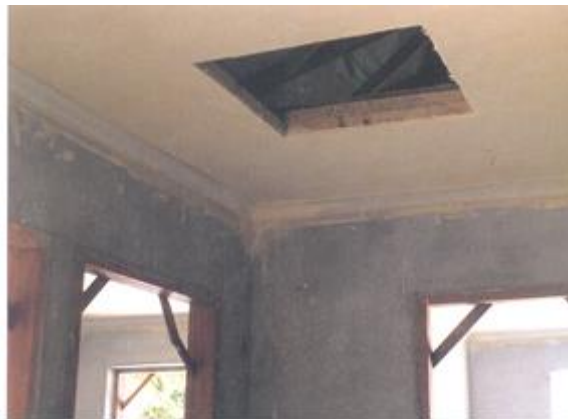
Figure 9.5 Newly erected plasterboard ceiling with access into the roof
