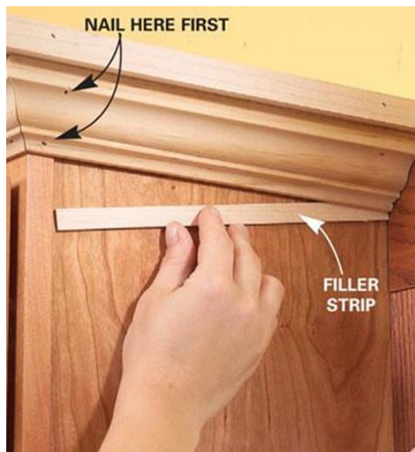
Figure 9.10 Adding a filler strip
